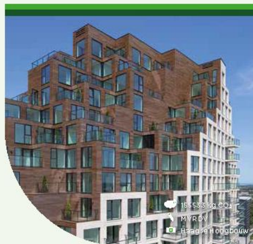
The Roofs residential towers Closed cladding installed at the crown of the buildings - (2200 m²) The Hague, the Netherlands
